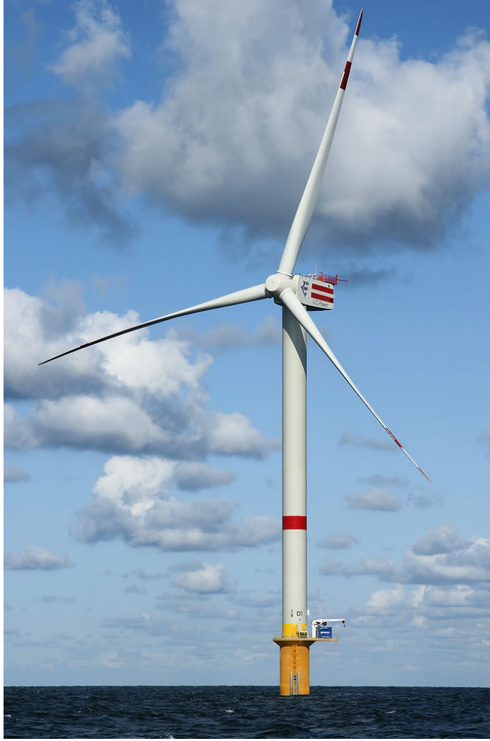
Figure 1.3: REpower 5M, with an output power of 5 MW and a rotor diameter of 126 m. Picture taken by Hans Hillewaert. Appendix B.
