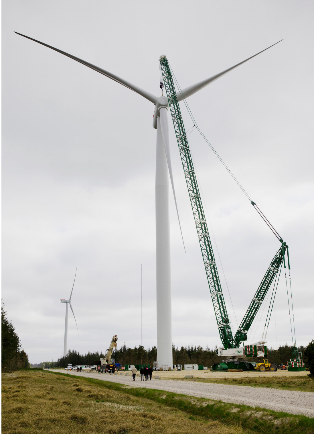
Figure 1.1: Siemens 7MW Wind turbine With a rotor diameter of 154 meters. (Photo: www.siemens.com/press , Appendix B)
